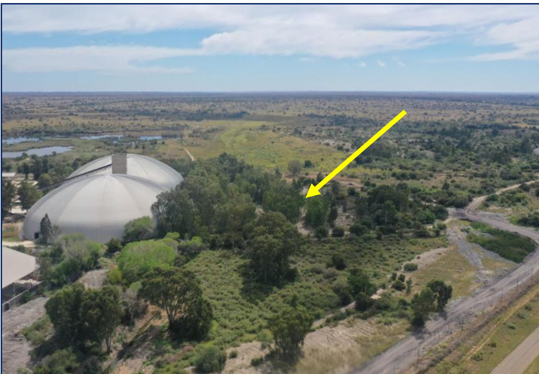
Plate 4: Oblique view of the area where infilling has been undertaken
